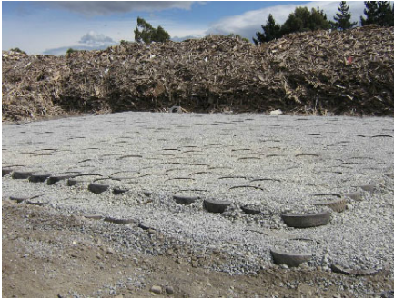
Ecoflex recycled tyre hardstand
