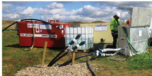
Heat exchanger captures heat from leachate
