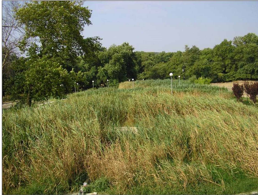
Figure 6. Typical view of a Constructed Wetland facility.
