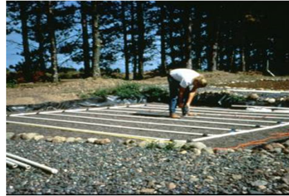
Drilled Manifold (orifices)
