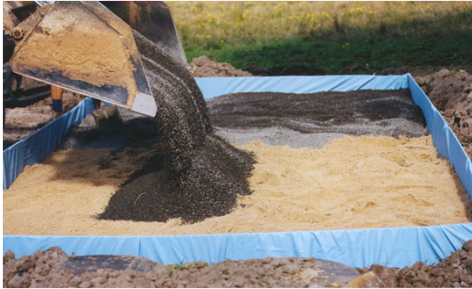
Filter sand and distribution bed
