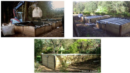
Peat Biofilter installation, VIC
