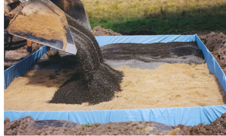
Filter sand and distribution bed
