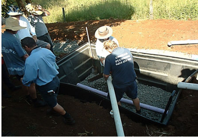
Underdrain and gravel bed
