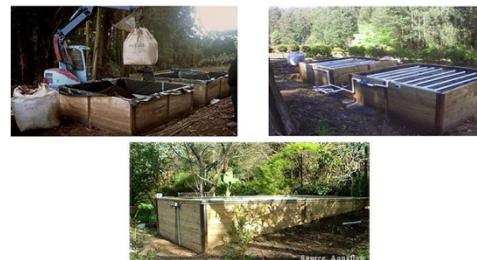
Peat Biofilter installation, VIC
