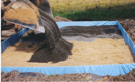
Filter sand and distribution bed
